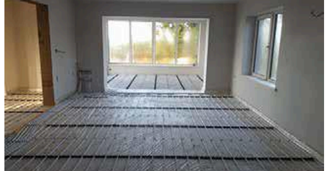
Extra fixings at bends and returns
