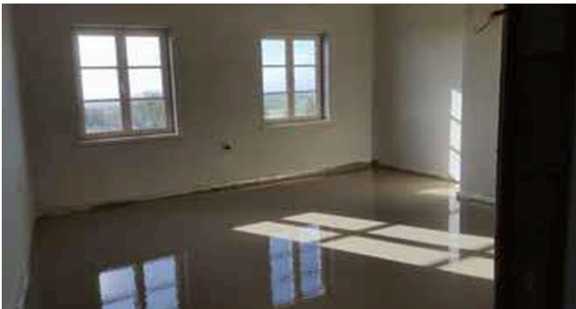
Screed placed to laser-set datum
