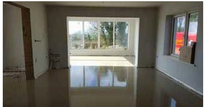
Level finish across the building
