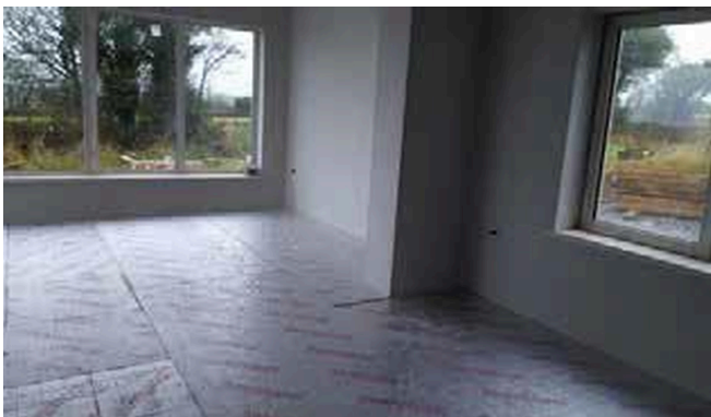
Membrane laid over the insulation
