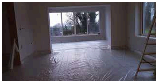
Ready for screed, no UFH
