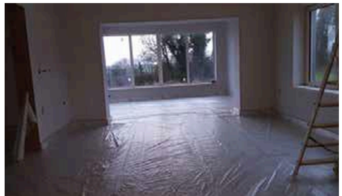
Joints taped, upturns returned up the walls
