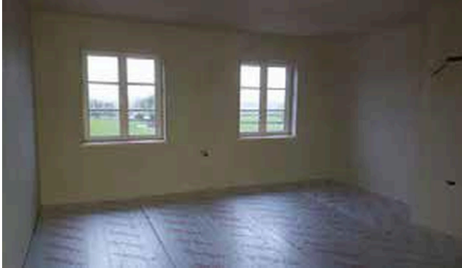
Insulation laid and edge strip fixed
