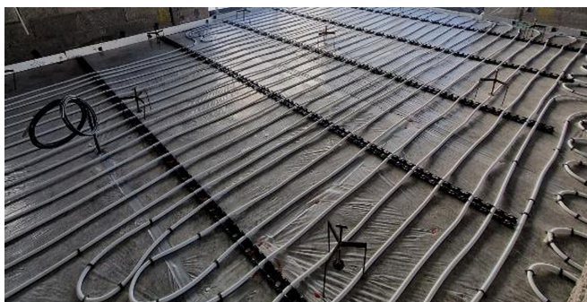
After UFH is laid
