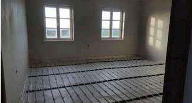
Pipes clipped at 500mm centres
